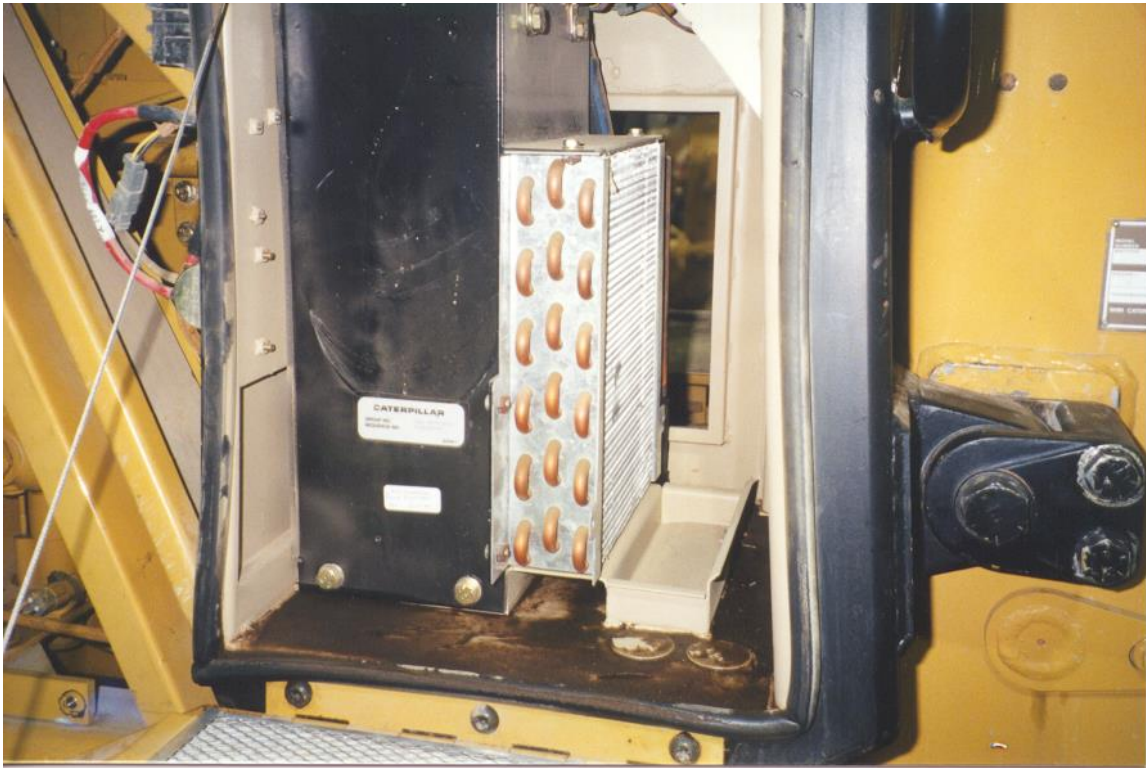
Heater area opened up for evaporator installation.
