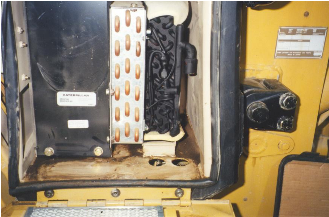
Evaporator in place against heater assembly.
